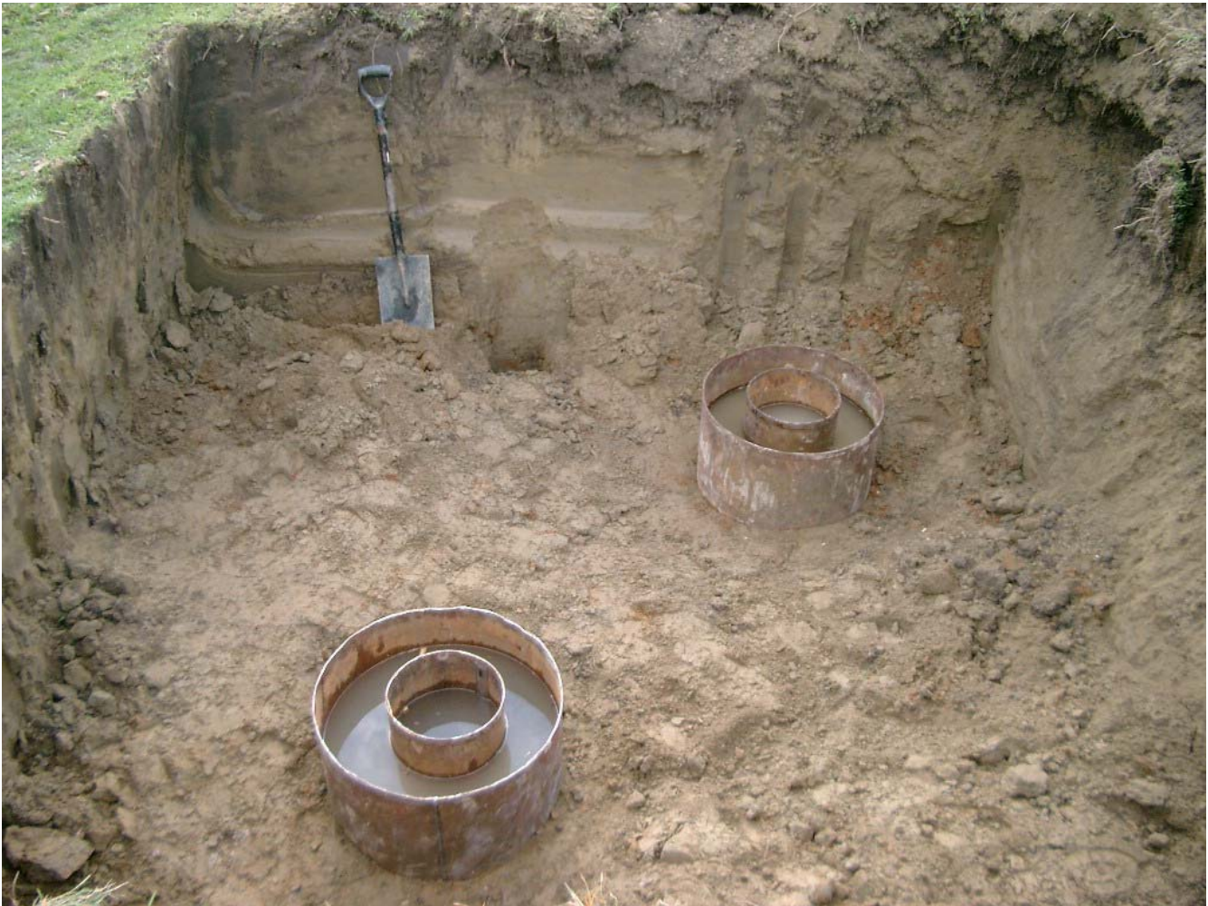
Photograph 1: Infiltration Testing of Sub-soils
