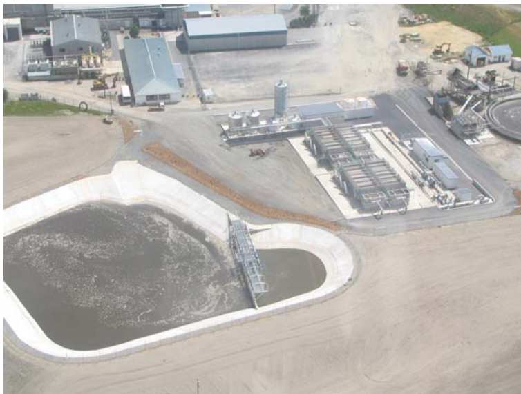
Photograph 1: Overall layout of the Finegand Upgraded Wastewater Treatment Plant
