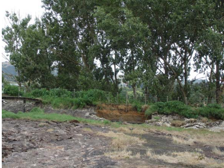
Photograph 4: Pond 1 Scarp on the inside Embankment
